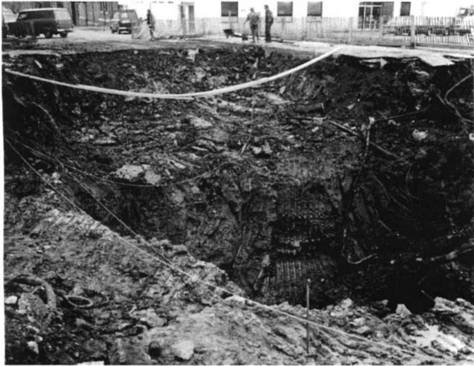
Figure 3.8(a) Four DDB collapse in Slone Street, Manchester – a few hours after collapse.
