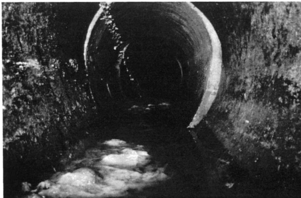
Figure 2.7 Typical egg-shaped clayware pipes in use.
