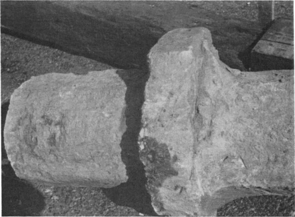
Figure 1.7 Section of limestone water mains with jointing collar recovered in 1983 from an excavation in Portland Street, Manchester – part of system of stone water mains laid between 1809 and 1813 by the Stone Pipe Company. The pipe is octagonal, 1 m long, with an external diameter of 0.8 m and an internal diameter 0.45 m.
