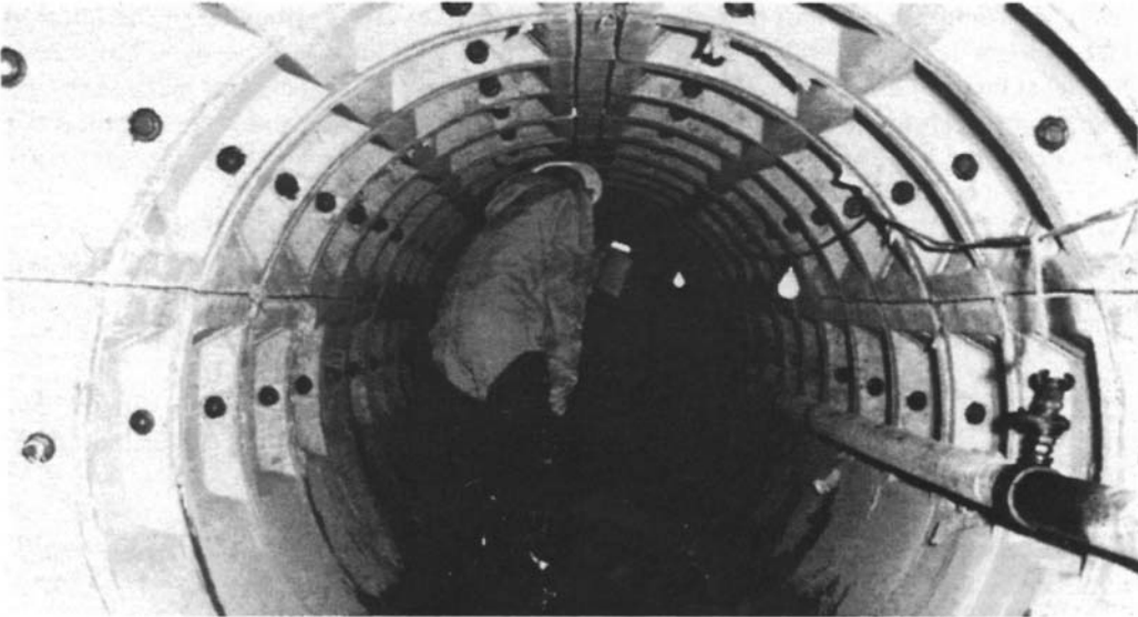
Figure 2.15 Sewer in concrete bolted segments, Market Street, Manchester.
