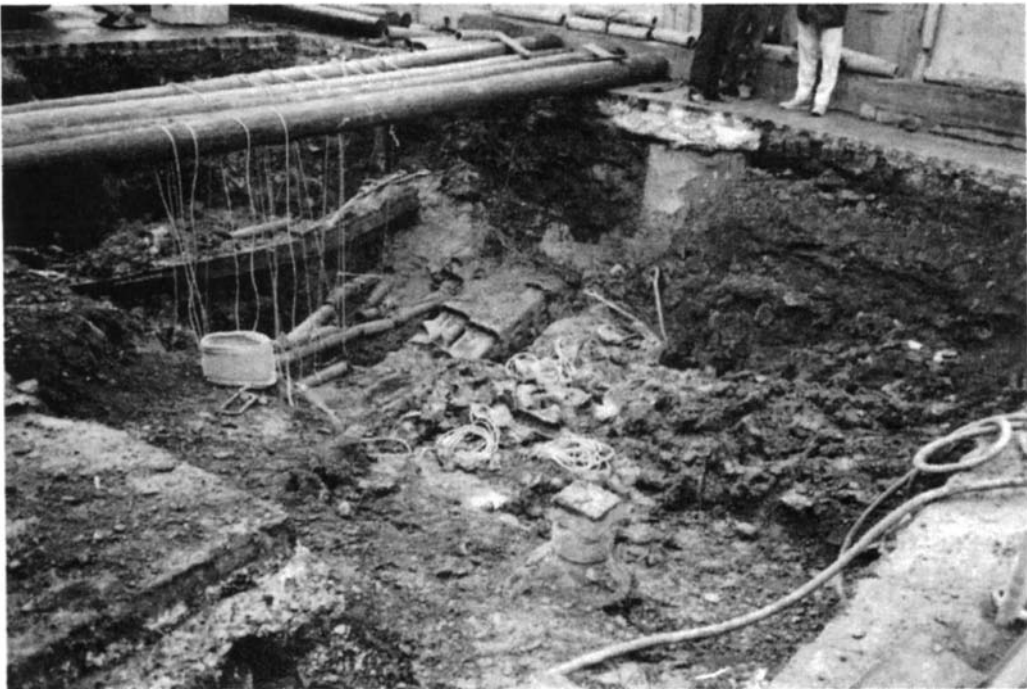
Figure 17.7(b) The offending cast-iron water main that fractured.
