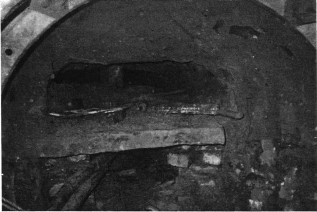
Figure 3.9 Original construction not properly backfilled.
