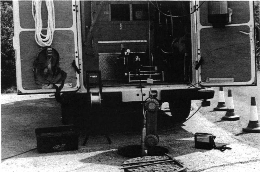
Figure 5.7 Back of survey vehicle showing camera being lowered into manhole. (Courtesy of Telespec Ltd.)
