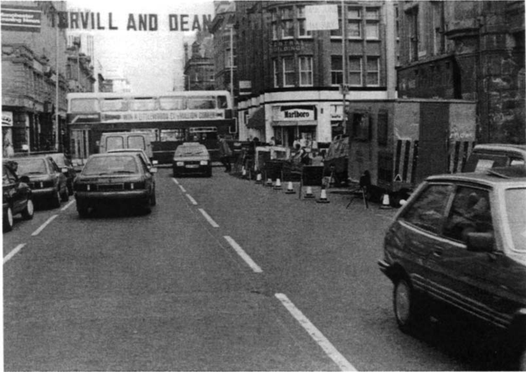
Figure 6.6 Traffic conditions in Deansgate once extent of cavity has been established, a few hours later.
