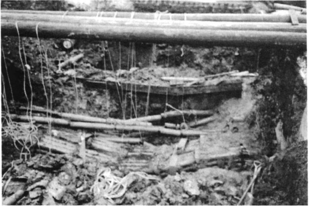
Figure 17.2 A large multiduct and other services (supported from above). The ducts had already sunk due to the sewer collapse.
