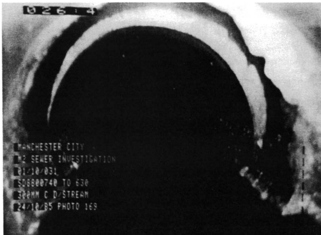
Figure 17.10 Detail of displaced joints.
