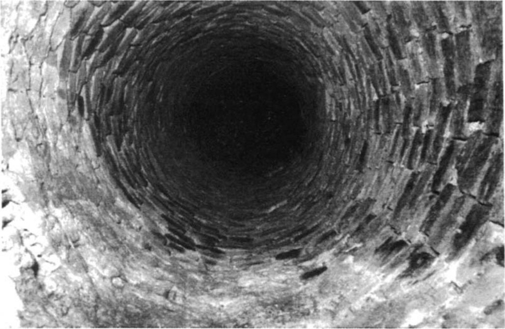
Figure 2.9 View of existing 'blind eye' shaft.
