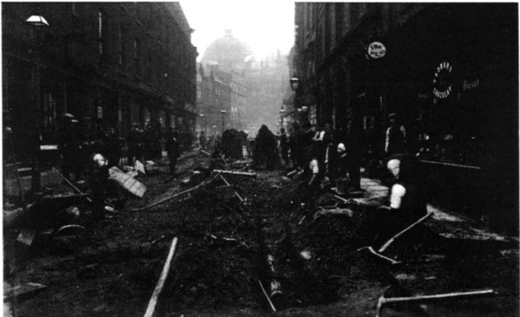
Figure 6.9 Old Millgate, Manchester, 1906.
