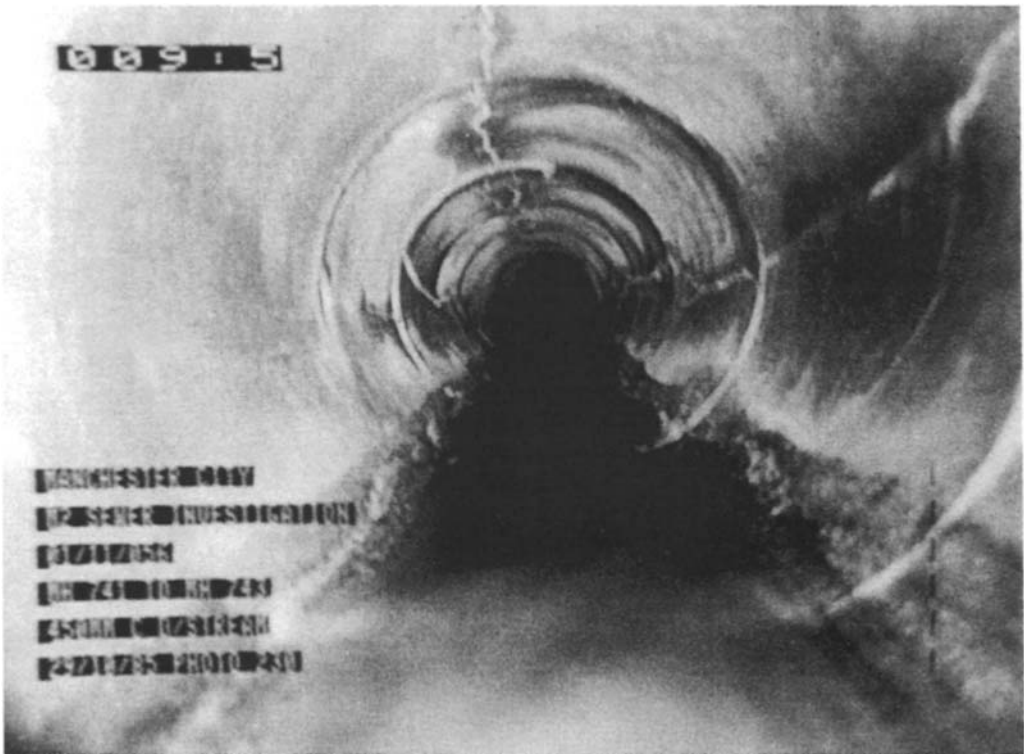
Figure 17.9 Detail of a cracked pipe.
