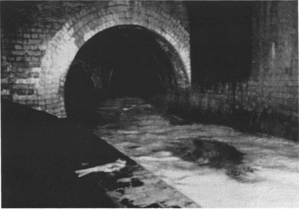
Figure 2.14 Junctions of work 5 and work 6, Rochdale Road, Manchester.
