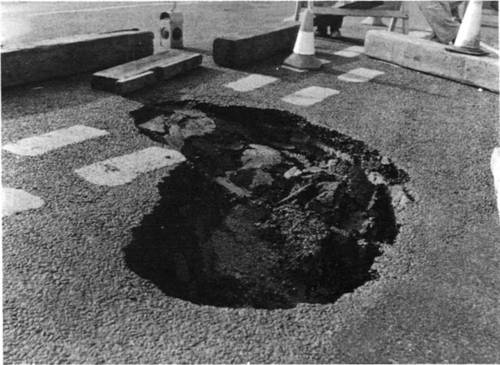
Figure 6.3 Surface evidence of sewer collapse.
