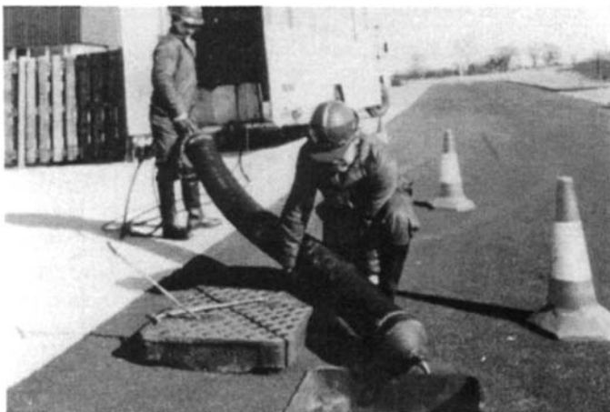
Figure 11.7 Inflatable packer assembly with integral resin injection head being lowered into a manhole.
