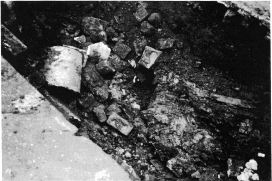
Figure 17.7(a) The beginning of the excavation onto the road depression.
