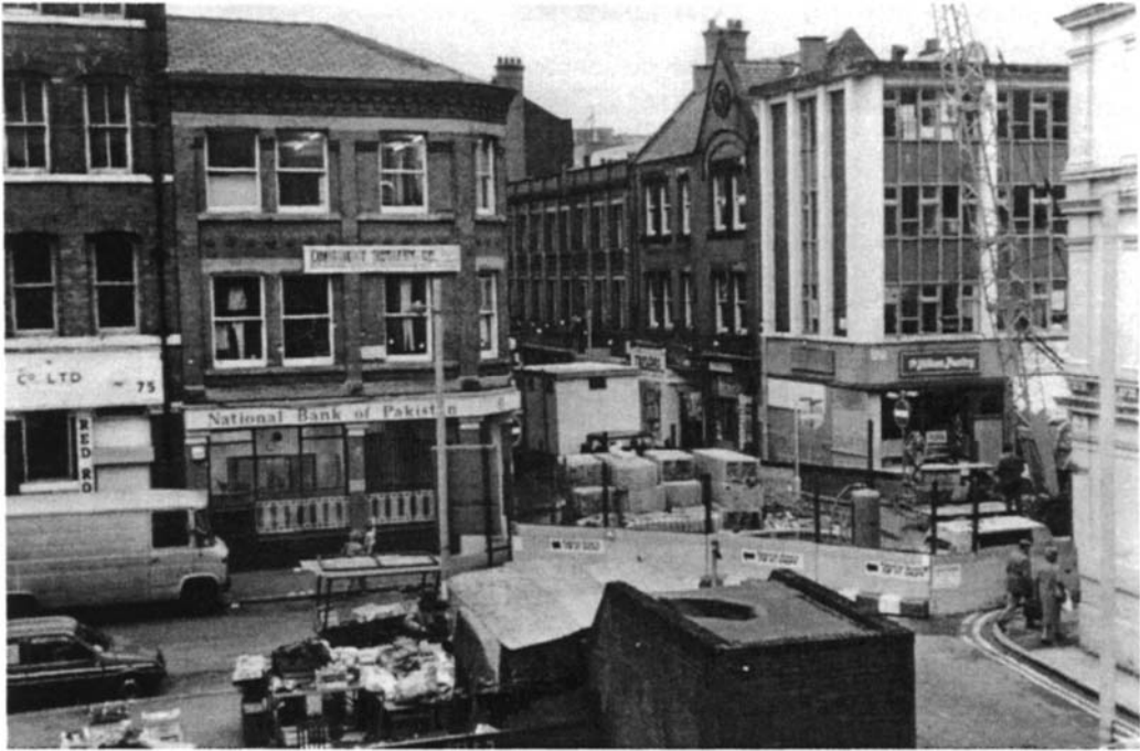
Figure 3.10 Construction of typical investigating shaft in city centre.
