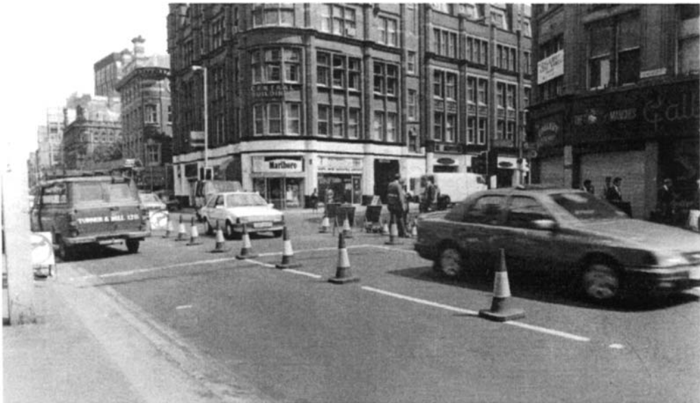
Figure 6.5 Traffic conditions immediately following the discovery of a sewer collapse in Deansgate, Manchester, 1990.
